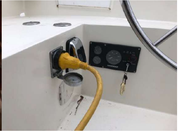
Vent, Pump, Engine Panel
